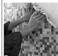
• Once the reference grid has been marked and the adhesive spread over the base, the laying begins by applying the mosaic sheet with the plastic film towards the operator and without exerting too much pressure.
