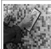
• Tap the mosaic with the rubber float to ensure perfect adhesion to the surface. During this operation it is possible to correct any errors that might have been made in the alignment by lightly tapping sideways on the sheets.
