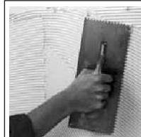
• To spread the adhesive use a toothed spatula (3 mm · 0.12" squared teeth). This spatula must be never used to hit or to move the laid sheets, as the metal, the glue and cement residual could damage the film.
